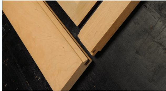
Dovetail construction
