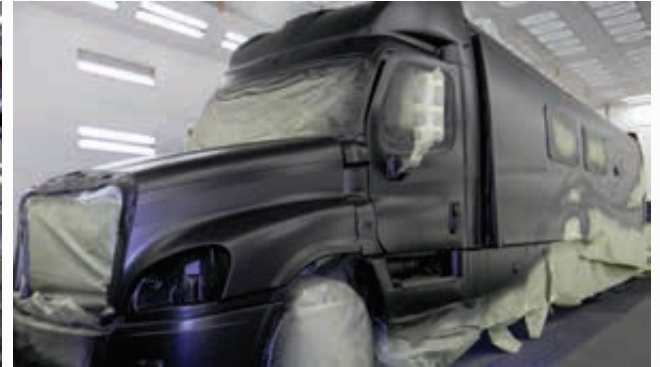
Black metallic base coat is applied.
