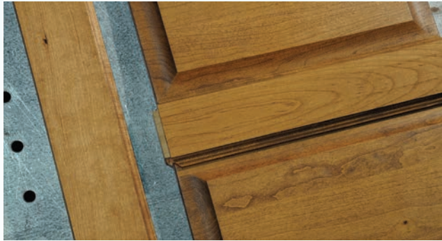
Raised panel door detail
