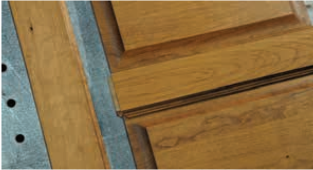
Raised panel door detail
