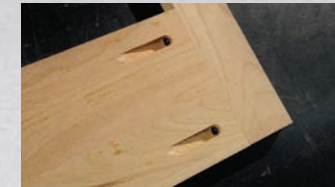
Pocket screws for structural integrity
